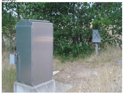
The large cabinet in front is apparently the control box for the UDOT traffic camera on top of a tall pole just out of sight to the left (see below). The smaller control box marked conveniently with an %+is what I had been looking for. UDOT must use the same data/audio link for both the camera and AM transmitter.
