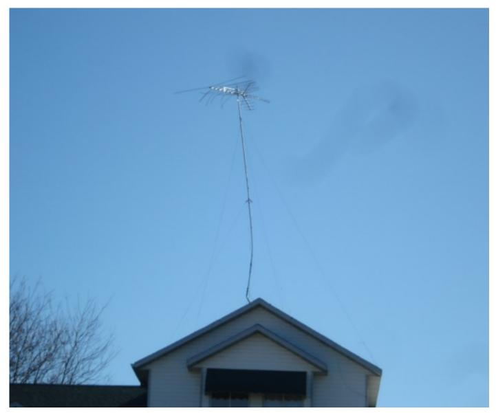
Over the years, I have admired professionally installed TV antennas. Most covered the old Very High Frequency (VHF channels 2 through 13) and Ultra High Frequency (UHF) TV channels (14 and up). The one shown above had the longer elements in the rear and were, of course VHF, and the shorter corner reflector elements at the front (pointing to the right toward Salt Lake City) were for UHF. Now that most all channels changed to UHF digital channels, the rear elements became less important.
